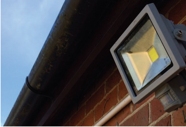
Poorly directed DIY floodlight (by Bob Mizon)
