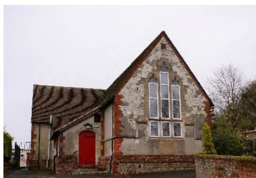
Figure 7.11: Grade II Former School, now village hall
