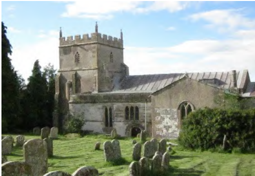
Figure 7.6: Grade I Church of St Mary
