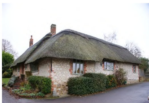
Figure 7.22: Unlisted The Old Stables
