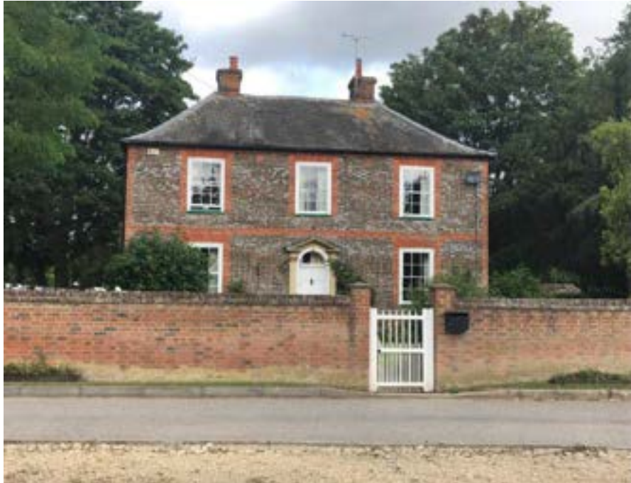
Figure 37. Listed building 18 th century farmhouse.
